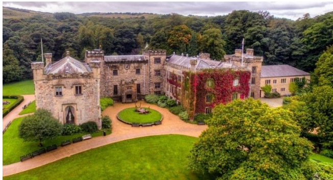
Visual grandeur of the building
